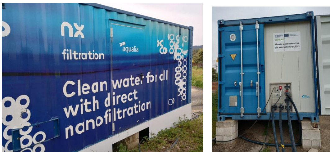
Figure 2. Nanofiltration pilot plant in Nogales DWTP (Badajoz, Spain)
