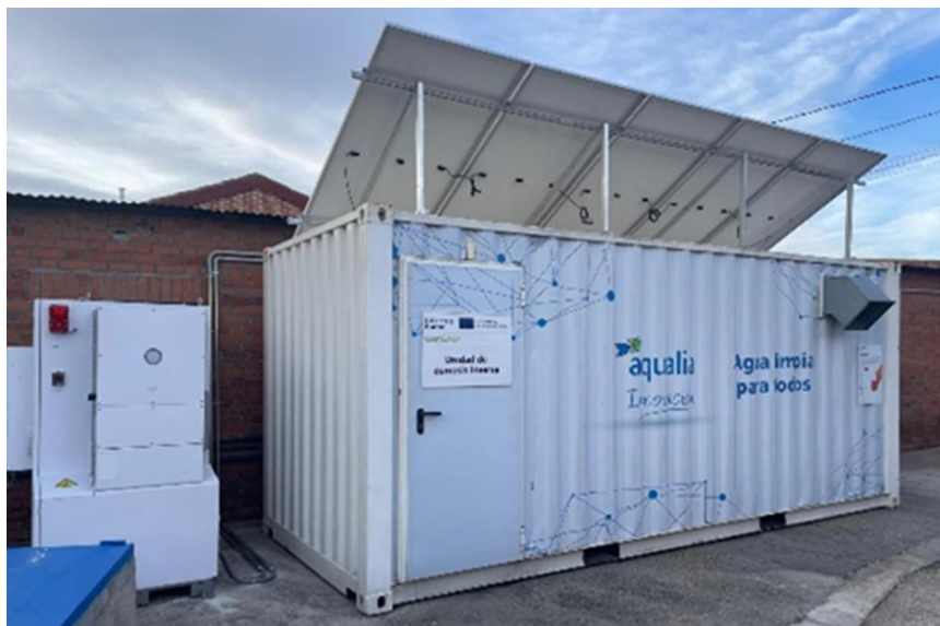
Figure 1. Reverse Osmosis pilot plant in Tiñosillos DWTP (Ávila, Spain)
