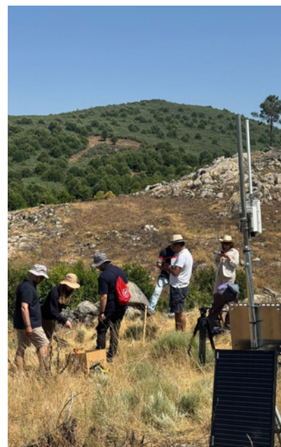
Installation of sensors within the deployment planned for 2025 for the early detection of forest fires.
